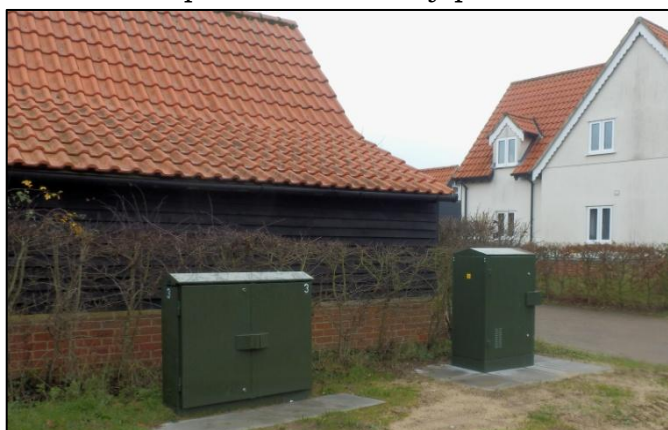
Fibre optics cabinets
