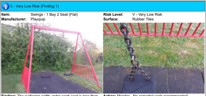
**Finding:** The surfacing width under each seat is less than **Action:** Monitor - No remedial work recommended 1.75 metres and fails the requirements of BS EN 1176 Part 2
