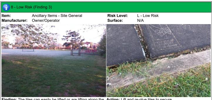
**Finding:** The tiles can easily be lifted or are lifting along the **Action:** Lift and re-glue tiles to secure edges of the area
