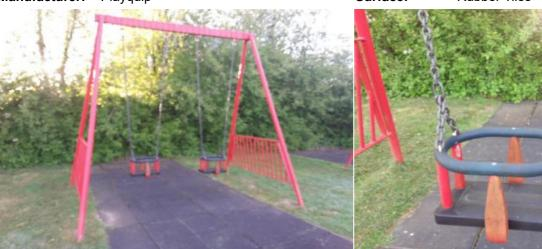
**Finding:** BS EN 1176 requires an additional 1.5m of unobstructed space at each end of the swing surfacing area. This is a relatively low risk finding and no remedial action is recommended at this point.
