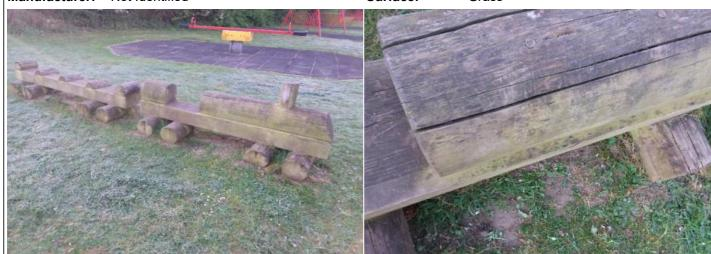
Finding: The timber has a number of splits/shakes or air cracks and this may affect the stability or allow water ingress fixing points of the structure and/or cause any instability which will accelerate the rotting process
