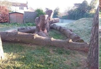
Finding: Due to the dimensions of the timber it was not possible to ascertain the condition of the timber at its core without further testing. We recommend a Resi-PD survey to establish the condition of the timber at it's core.
